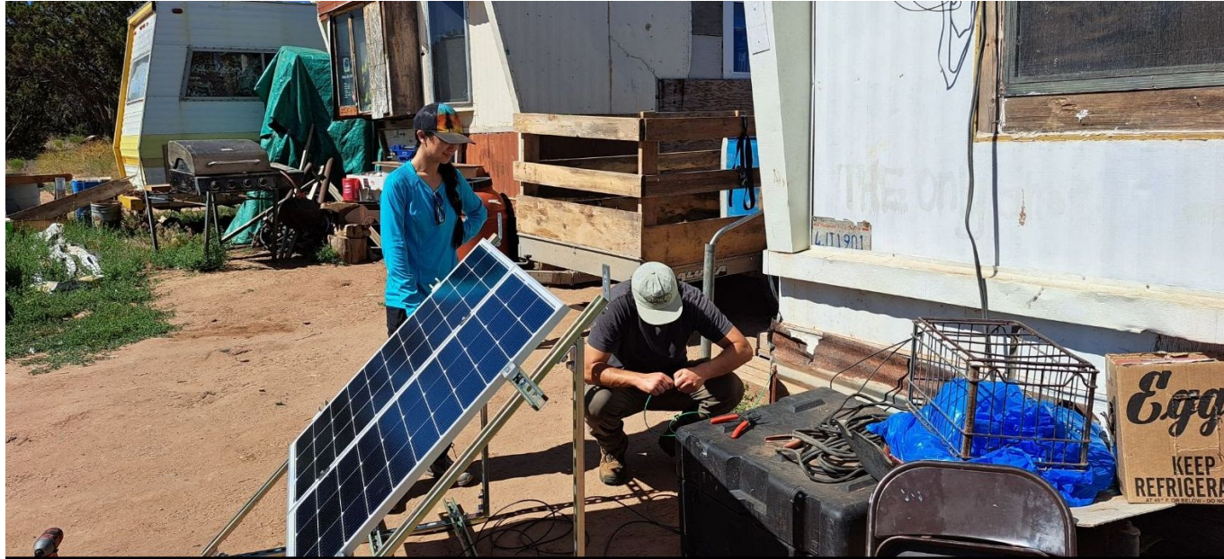
Attaching the frame grounding wire
