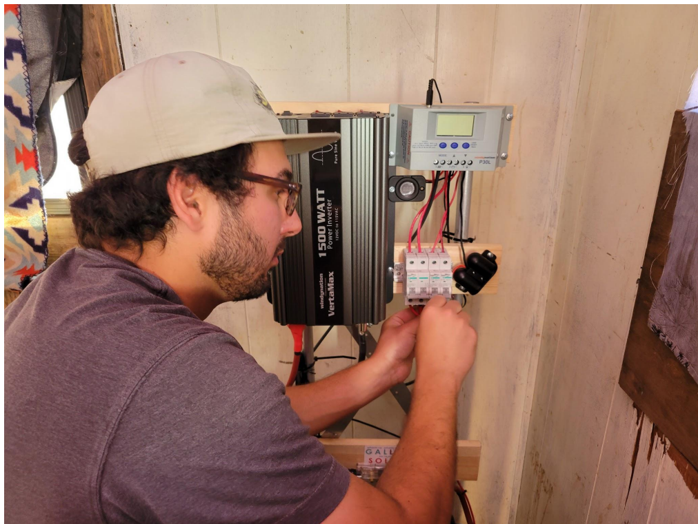
Connecting the PV wires to the circuit breakers
